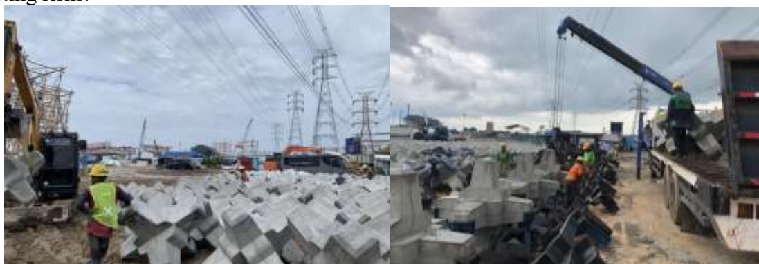
Figure 2. Observation of the Construction and Mobilization Process of the Armor Jack
